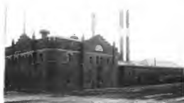
PUMPING STATION, YOUNGSTOWN
